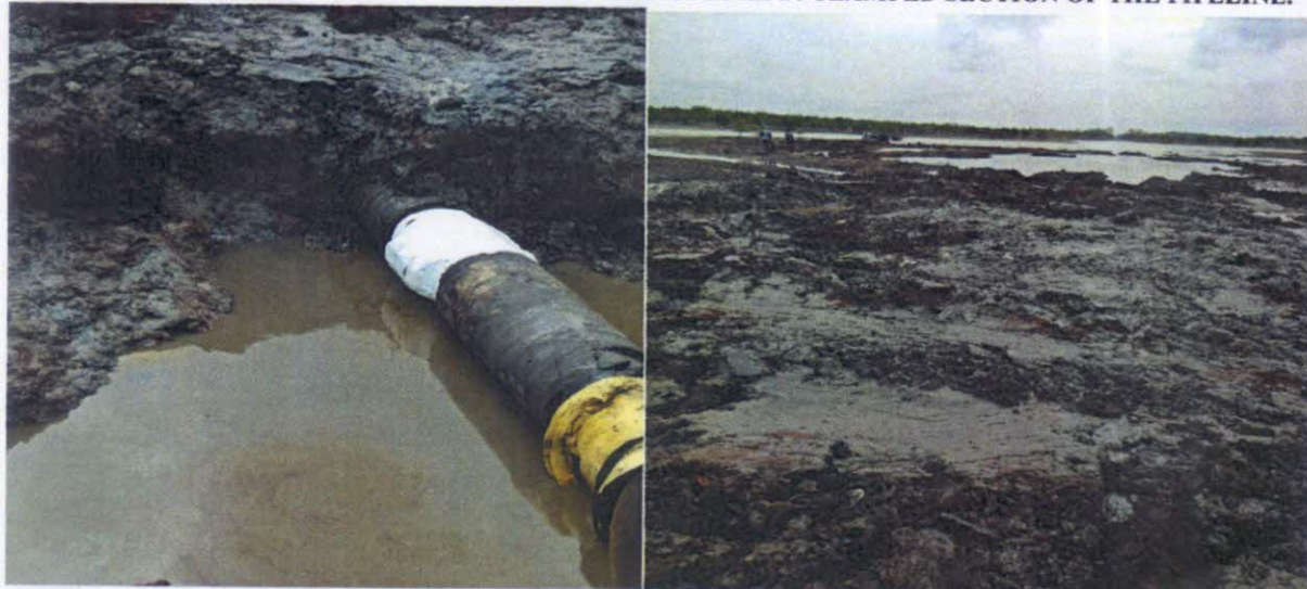
PICTURE C: REPAIRED SECTION AFTER WRAPPING. PICTURE D: INCIDENT POINT AFTER BACKFILLING.
